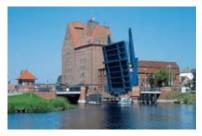
Traffic in/on the crossing routes is either released or blocked. The mobile superstructure/the mobile superstructure component is designed as a bascule, swing or lift bridge, i.e. rotated on a horizontal or vertical axis or lifted vertically on lifting towers.
