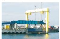
Consequently, ferry terminals are the landside connecting constructions to ferryboats and bear railway tracks (traject bridges), roadways or paths (e.g. Ro-Ro bridges) with the same elements of technical equipment.
